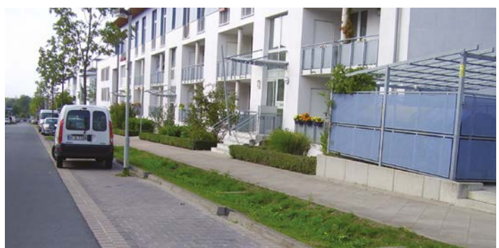
Stormwater infiltration below a public parking area.
